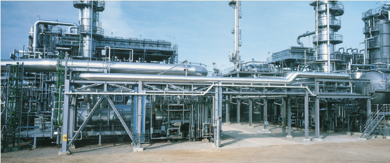
FIGURE 2: A Claus unit of a major German oil refinery, which is used for the recovery of sulfur from hydrogen sulfide, is used as a case study in the FEE project.
